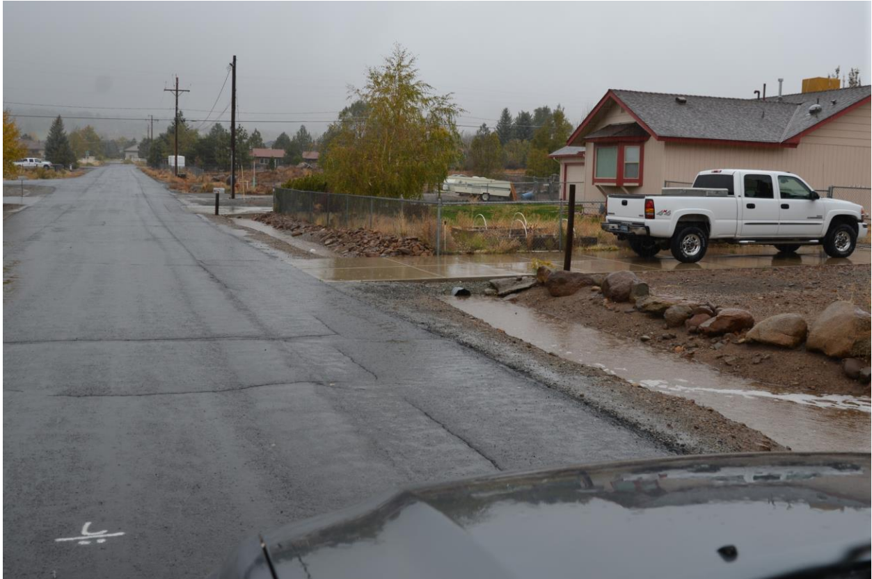
Photograph 3. Storm water drainage on Shawna Lane. Photograph Taken on 10/16/2016 2:01 P.M.
